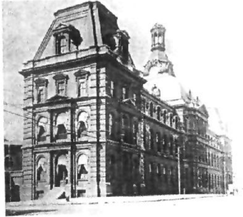
THE FOUR COURTS BUILDING
